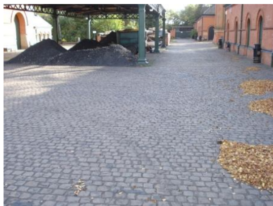
Cobbles around the Boiler House
